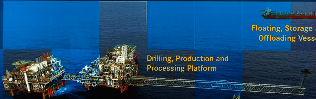
Compression, Utilities and Quarters Platform
