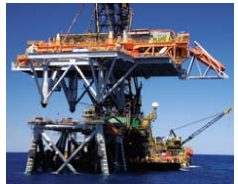
▲ A topside module is lifted onto the jacket.
